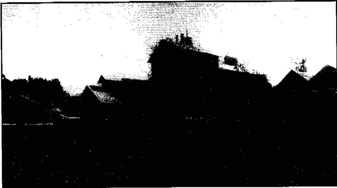
The core buildings of the ironworks shown in a photograph probably taken after 1903 when the furnace ceased operations. The blast furnace was enclosed in the tall building at the center. The casting shed is the low building to the left with the ridge ventilator. The engine house with the blowing tubs is on the far left. The charcoal storage sheds are located on the hilltop to the right.
