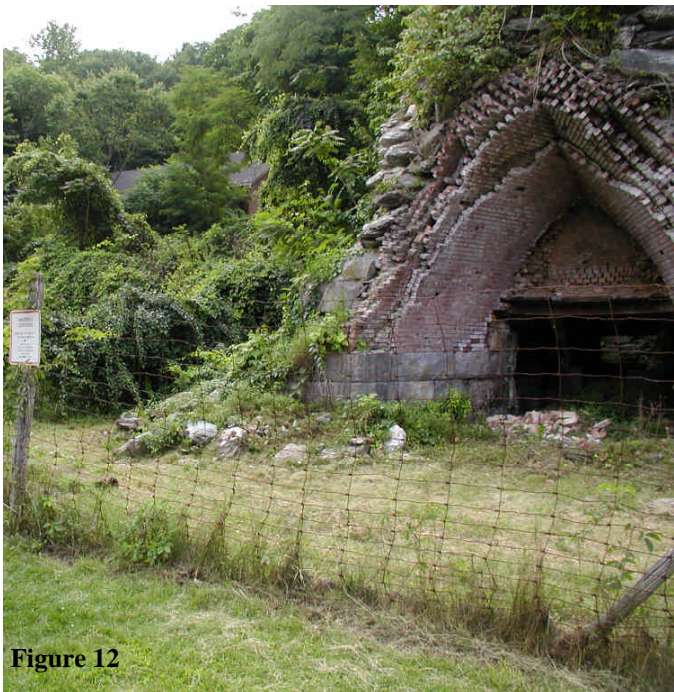
Figure 12: Recent image of furnace showing progressive deterioration. Note the extensive plant growth and collapsed masonry surrounding the foundation.
